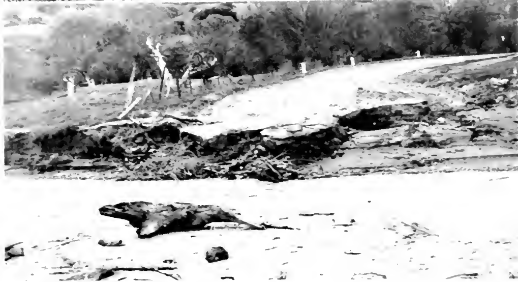
Above—"Sea-going" bridge anchored by cable. Below—Typical road washout
